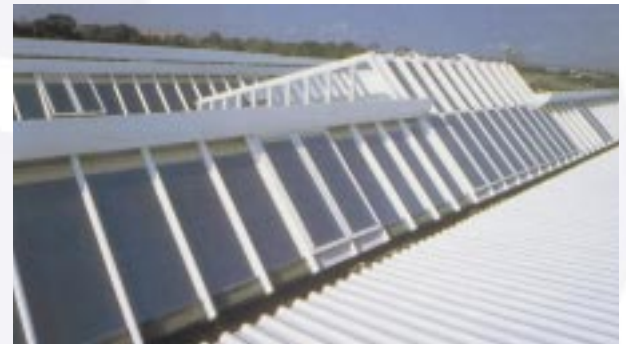
A typical exterior application of Designer Series film to rooflights
