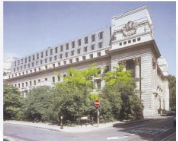
Madico Protekt Neutralux 100 micron combined solar/safety film to Grade 2 listed building
